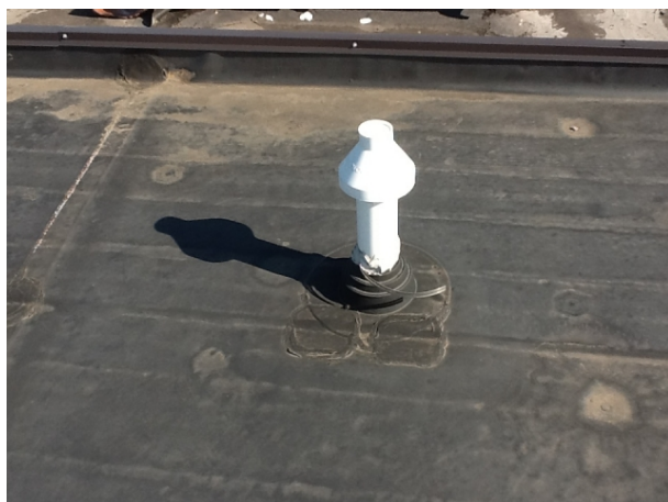
Typical pipe penetration 2 located on office roof area
