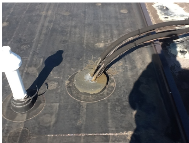
Typical Line Set flashing 1-located on office roof area
