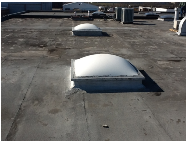
Typical Skylight 4-3x3 skylights on Front Shop Roof Area
