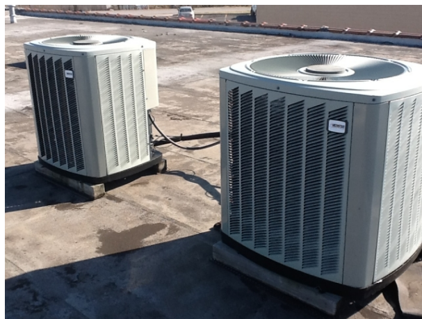
Typical Condensors 2-located on Front Shop Roof Area
