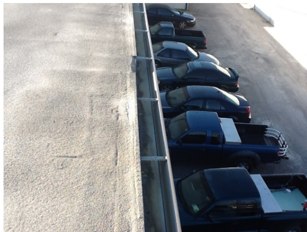
Guttered Edge Approx 60 LF along North side of Roof Area
