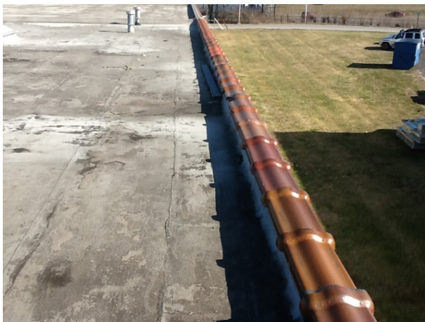
Clay coping cap Approx 60 LF @ South wall
